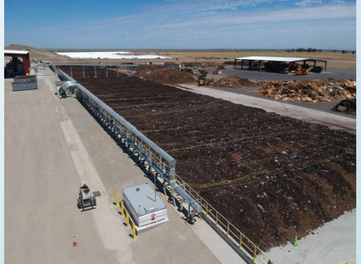
Covered aerated static pile system at Yolo County Central Landfill
